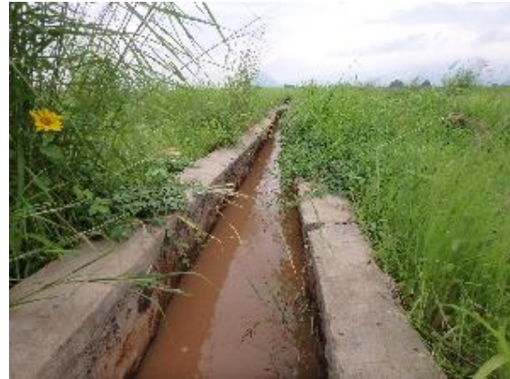
Masonry retaining wall canal (Msagali, Mpwapwa, Central)
